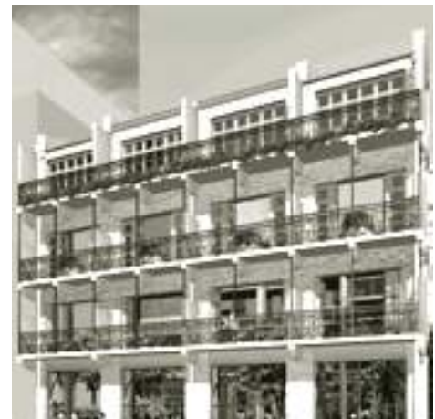
Plate 4: After revitalisation - Mallory Street/Burrows Street Project, Wan Chai
