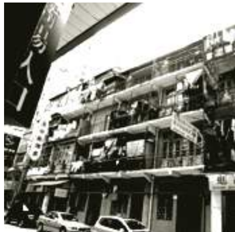
Plate 3: Before revitalisation - Mallory Street/Burrows Street Project, Wan Chai
